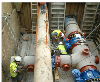
SIERG – GRENOBLE (38) AEP BETON ÂME TOLE Ø 800 TRAM
